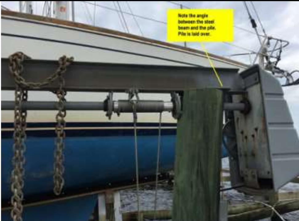
Note the angle between the steel beam and the pile. Pile is laid over.
