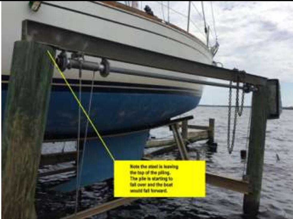
Note the steel is leaving the top of the piling. The pile is starting to fall over and the boat would fall forward.
