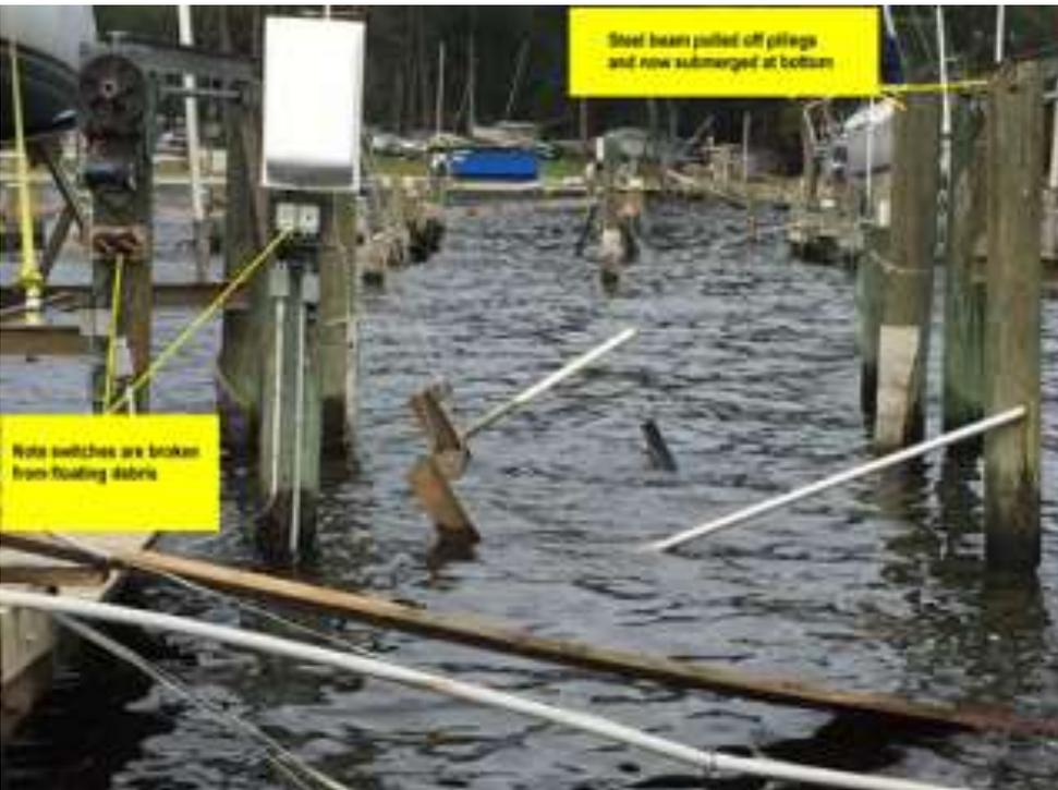
Steel beam pulled off pilings and now submerged at bottom
